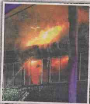
The building ablaze.
