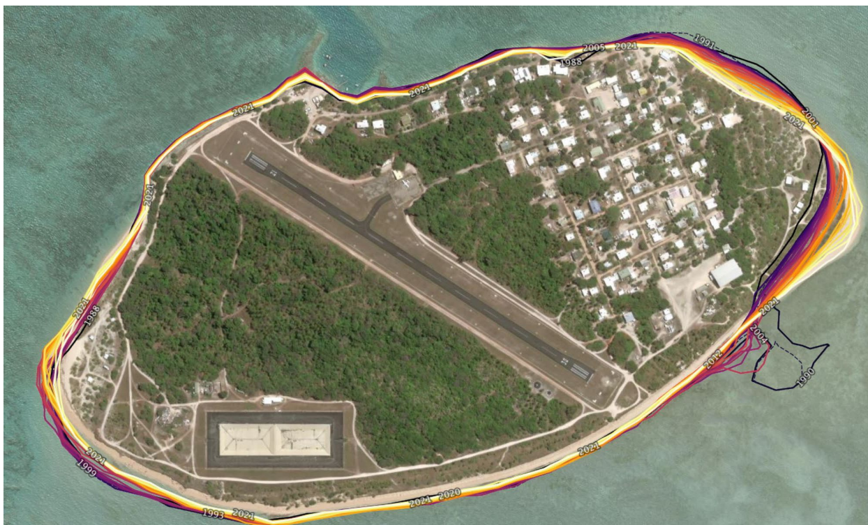
Figure 39 Satellite images over the last 30 years reveal that Warraber's eastern and western ends are experiencing erosion and accretion, with beach rock stabilising the north coast.
